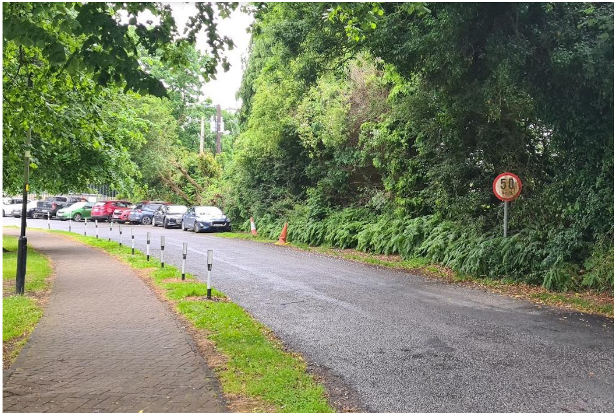
Figure 8 – Existing Posted Speed Limit
